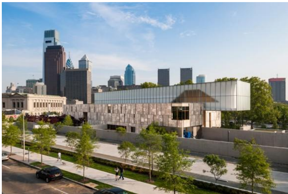
Outside the Barnes Foundation in Philadelphia. Photo: Tom Crane/Barnes Foundation.
